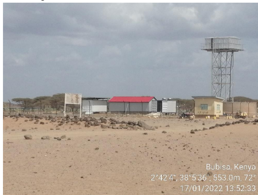
Figure 19: Bubisa Water Desalination Plant
