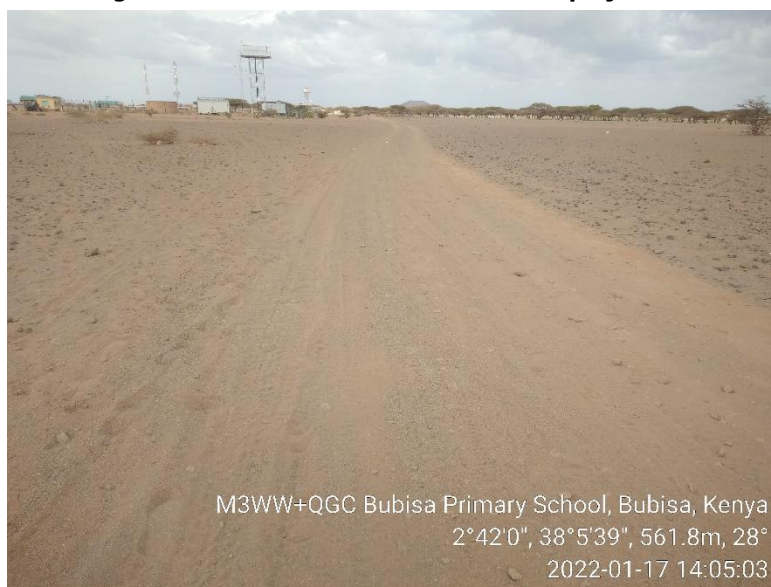
Figure 20: State of the access road to the project site
